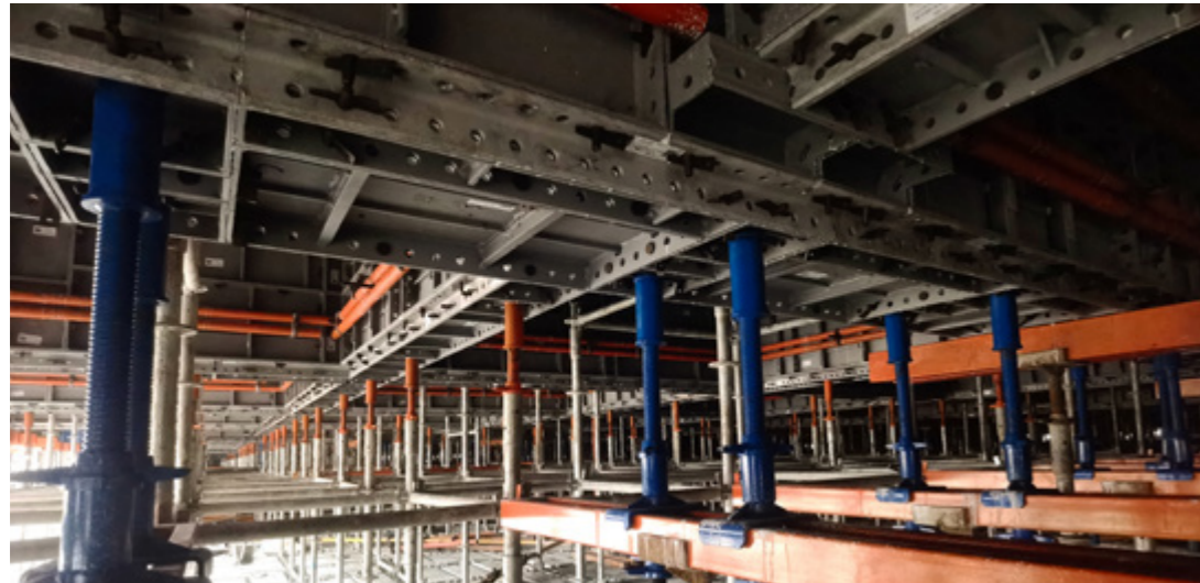
Early-removal Node Scheme for Main Beam 主梁早拆节点方案
