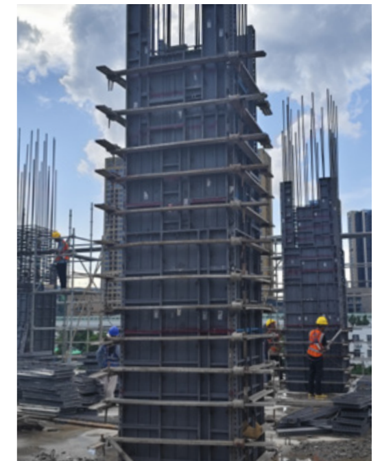
Column Formwork Solution 2
