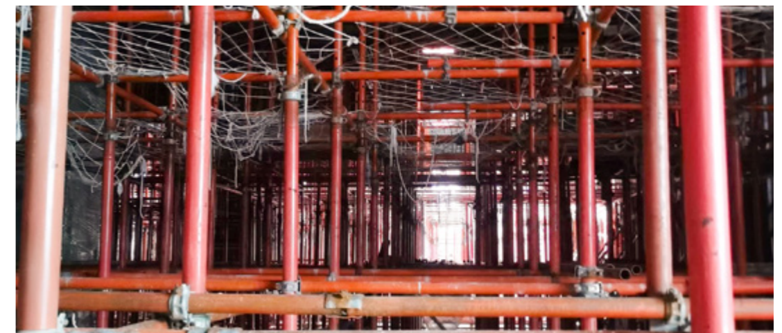
Construction Method of Independent Support and Aluminium Formwork 独立支撑 + 铝模施工工艺
