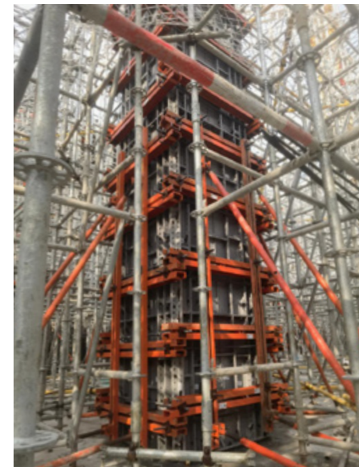
Column Formwork Solution 1
