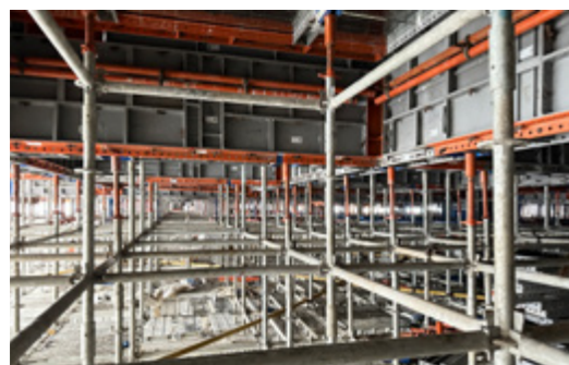
Early-removal Node Scheme for Main Beam 主梁早拆节点方案
