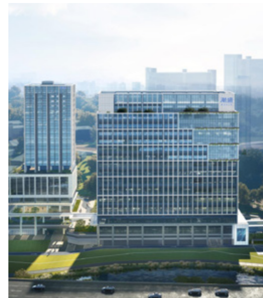
ChaoSheng Building 潮盛大厦
